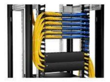
A patch panel is a device or unit in which many sockets are generally similar or same. They can be used in a convenient way for the use of connection and a routing circuits for connections, texting of circuits and monitoring. They are designed to be flexible. Patch panels are deeply used in computer networks, radio, T V and recording studios.
