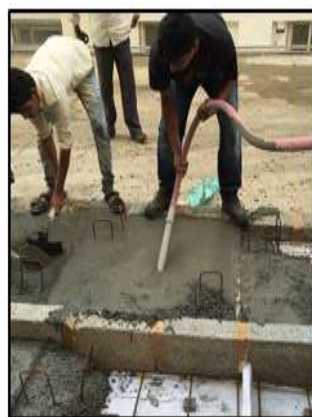
Fig.6: Pouring and vibrating of concrete
