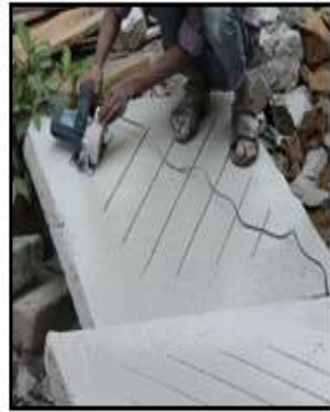
Fig 12: Groove Cutting
