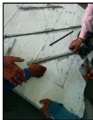
Fig 15: Placing of Strips
