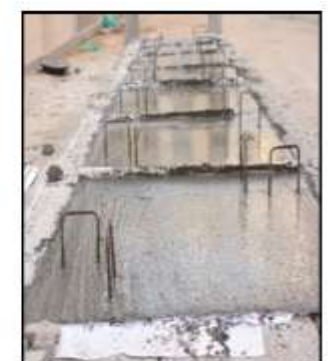
Fig.10: Finishing of placed concrete
