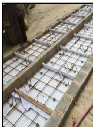
Fig.5: Reinforcement in the mould.
