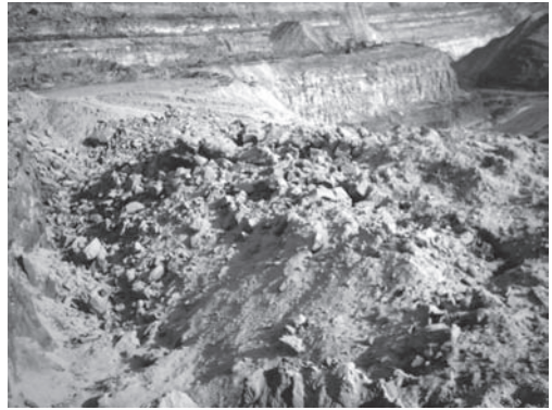
Figure 10. Plate showing blasted muck after side cast blasting at site.
