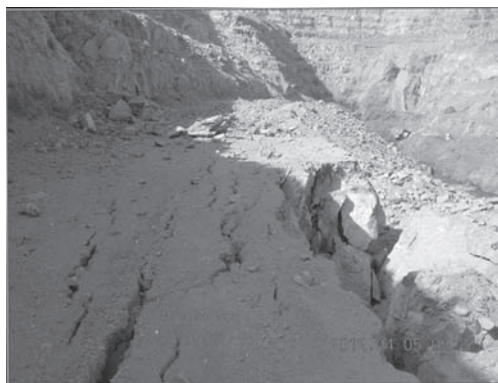
Figure 4. Failure pattern showing opening of foliation planes.
