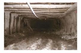
Figure 2. An example of rectangular roof bolted roadway in one of U.S. mines.
