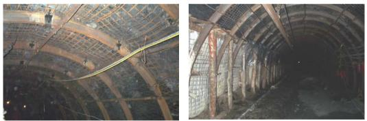
Figure 6. Reinforcement of steel yielding arches in gateroads by means of: (a) bolting cross bar arches with fully resin steel bolts, (b) roadside pack of mineral binding material.
