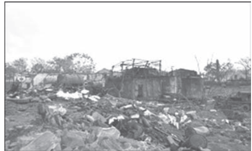
Figure 2. Damage industrial areas.
