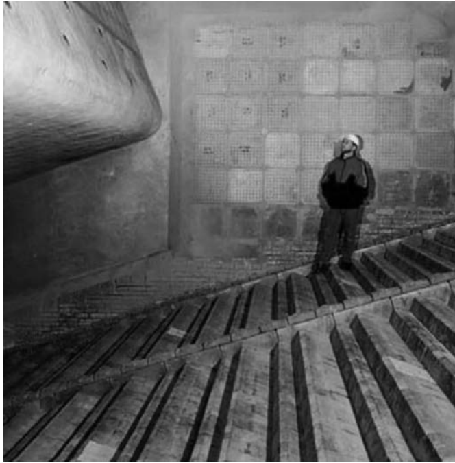
FIGURE 8.11 Reciprocating grate showing protective refractory sidewall. (Courtesy of Von Roll Inova, Ltd.)
